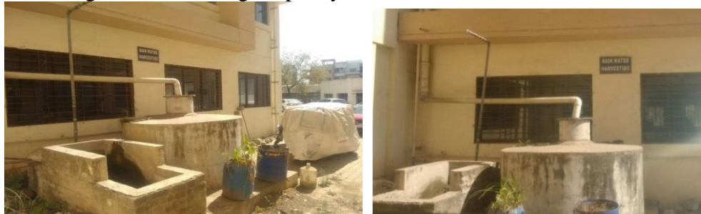
Fig.7.3 Rainwater Harvesting System
